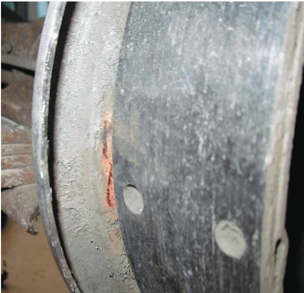
Figure 18. Rusty and worn backing plate.
