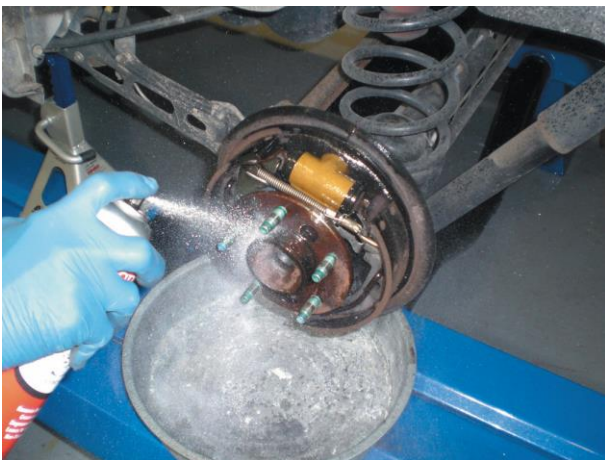
Figure 15. Wet down the assembly to trap any dust that may contain asbestos.
