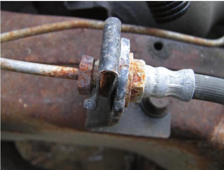
Figure 32. Check for leaks at hydraulic system fittings.
