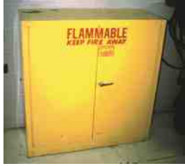
FIGURE 7.6 Typical fireproof flammable storage cabinet.
