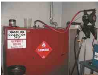
FIGURE 7.4 A typical aboveground oil storage tank.
