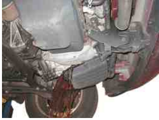
FIGURE 69.6 Draining the fluid from an automatic transaxle by allowing the fluid to flow into a container after most of the retaining bolts have been removed.
