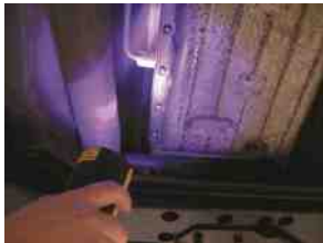
FIGURE 69.5 A black light being used to locate the source of an automatic transmission fluid leak.
