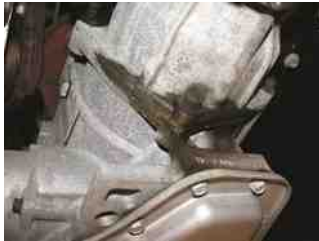
FIGURE 69.4 Sometimes the location of a transmission fluid leak is easy to see, but with others it can be difficult to find the exact location. Look closely at places where O-rings or gaskets are used, as these are the most common areas where fluid leaks occur.
