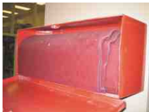
FIGURE 6.14 A treated wool blanket is kept in this easy-to-open wall-mounted holder and should be placed in a centralized location in the shop.
