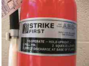
FIGURE 6.12 A typical fire extinguisher designed to be used on type class A, B, or C fires.
