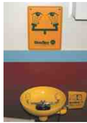
FIGURE 6.16 A typical eye wash station. Often a thorough flushing of the eyes with water is the best treatment in the event of eye contamination.
