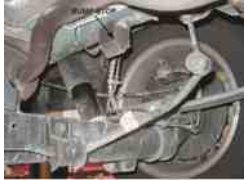
FIGURE 49.18 Carefully inspect the bump stops for damage during a thorough visual inspection.
