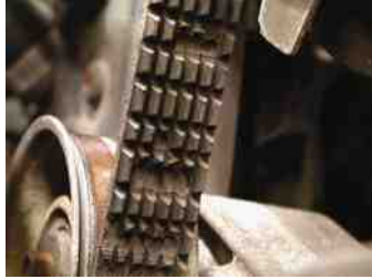
FIGURE 31.6 This accessory drive belt is worn and requires replacement. Newer belts are made from ethylene propylene diene monomer (EPDM). This rubber does not crack like older belts and may not show wear even though the ribs do wear and can cause slippage.
