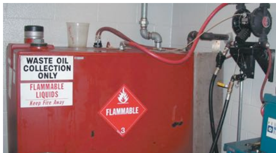
Figure 2-4 A typical aboveground oil storage tank.
