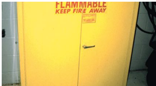
Figure 2-6 Typical fireproof flammable storage cabinet.
