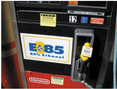
FIGURE 6-5 A pump for E85 (85% ethanol and 15% gasoline). E85 is available in more locations every year.
