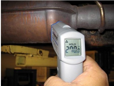
FIGURE 28-11 The temperature of the outlet should be at least 10% hotter than the temperature of the inlet. If a converter is not working, the inlet temperature will be hotter than the outlet temperature.
