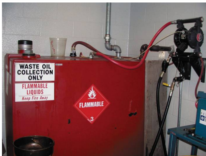
FIGURE 2-3 A typical aboveground oil storage tank.
