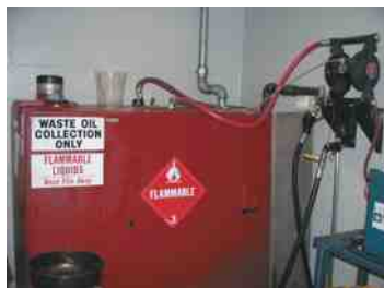
FIGURE 2-3 A typical aboveground oil storage tank.
