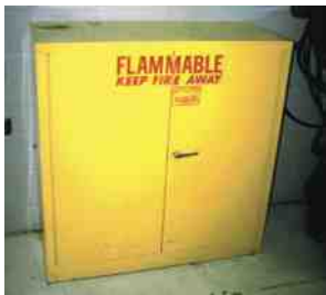
FIGURE 2-5 Typical fireproof flammable storage cabinet.
