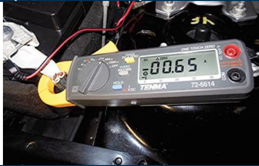
FIGURE 6-17 Clamp-on digital multimeter (DMM) used to check battery electrical drain. Meter reads over a half an ampere, which exceeds normal specification of 0.050A.
