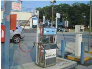
FIGURE 6-14 This CNG pump is capable of supplying compressed natural gas at either 3,000 PSI or 3,600 PSI. The price per gallon is higher for the higher pressure.
