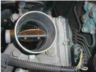
FIGURE 29-11 The throttle plate stayed where it was moved, which indicates that there is a problem with the electronic throttle body control assembly.
