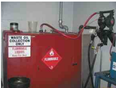
FIGURE 2-3 A typical aboveground oil storage tank.
