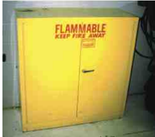
FIGURE 2-5 Typical fireproof flammable storage cabinet.
