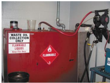
FIGURE 2-4 A typical aboveground oil storage tank.
