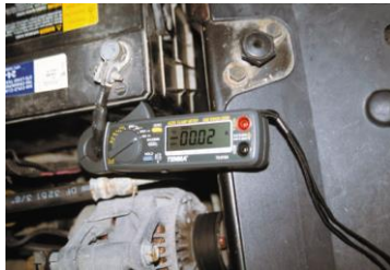
FIGURE 17-14 This mini clamp-on DMM is being used to measure the amount of battery electrical drain that is present. In this case, a reading of 20 mA (displayed on the meter as 00.02 A) is within the normal range of 20 to 30 mA. Be sure to clamp around all of the positive battery cables or all of the negative battery cables, whichever is easiest to clamp.
