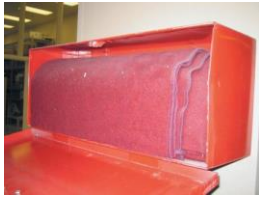
FIGURE 1-14 A treated wool blanket is kept in this easy-to-open wall-mounted holder and should be placed in a centralized location in the shop.
