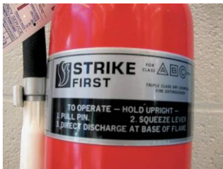
FIGURE 1–12 A typical fire extinguisher designed to be used on type class A, B, or C fires.
